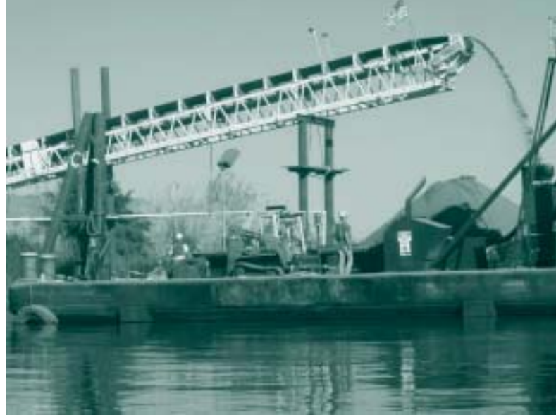
Above: During Phase II, 270,000 yards of material was removed from Decker Island and used to rehabilitate other islands' levees.
