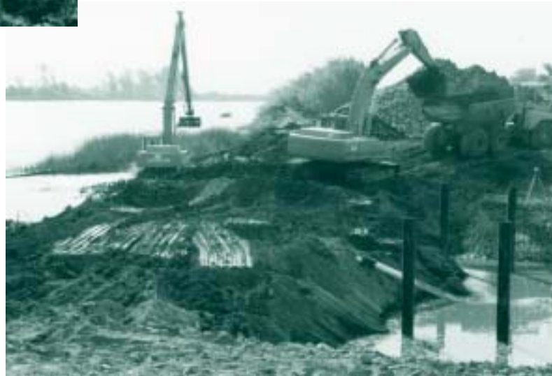
Below: A breach was created to allow the Sacramento River to flow into the awaiting wetlands.
