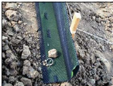
Side view: staked, not yet backfilled
