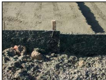
Stakes on downstream side
