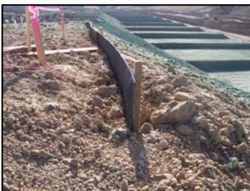
Side view—trenched, backfilled and staked
