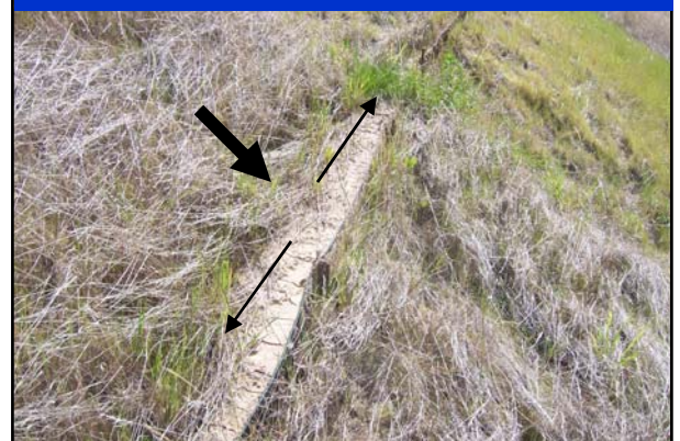
ProWattle tends to spread concentrated flow into sheet flows—reducing the chances of erosion damage
