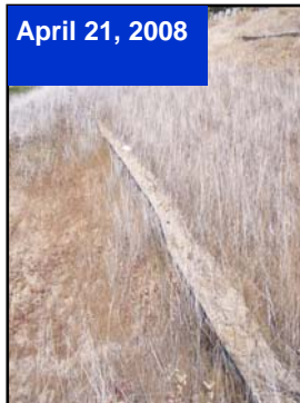
ProWattle tends to spread concentrated flow into sheet flows—reducing the chances of erosion damage
