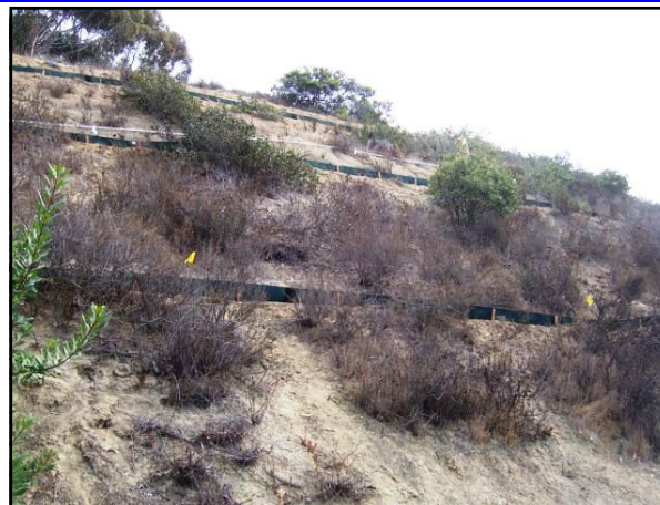
PW was installed on steep slopes throughout SIO
