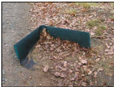
Velocity check for ditch or channel
