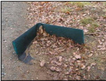
Velocity check for swale or channel
