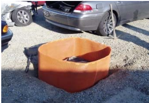
Installation in progress: Prior to stakes and backfill
