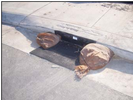
Anchored with Gravel Bags
