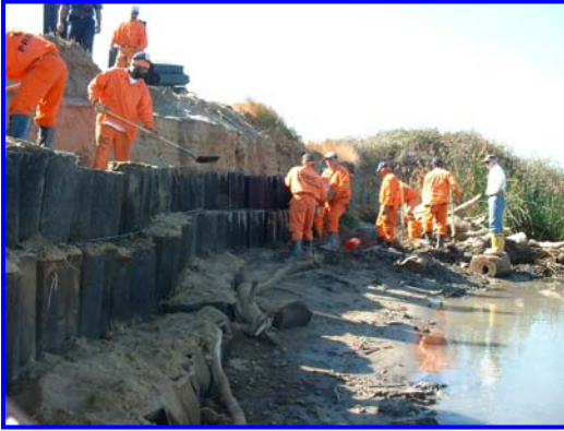
Figure 3: Installation in progress
