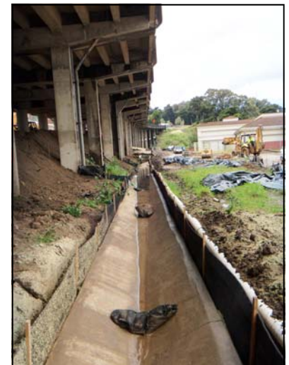
S-Fence 20" installed on both sides of concrete V-Ditch
